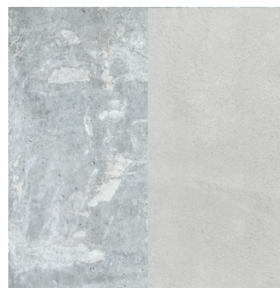
laitance removal before and after
